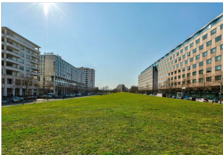
Park right outside the building
